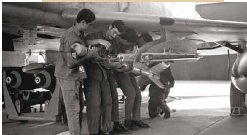
During the first weeks of the War of Attrition ground crews were able to gain substantial experience in arming and unarming their aircraft. In the top picture M117 bombs receive their fuses shortly prior to a bombing mission, while in the photograph below four airmen load a 90 kg heavy AIM-9D, IAF code Dekker (Rapier), on the left inboard pylon of a Kurnass.
